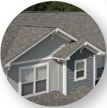
Roofing and Ventilation
